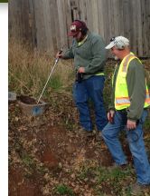
PCWA staff utilizing a ground microphone to listen for leak sounds with supervision from USA Trainer.
